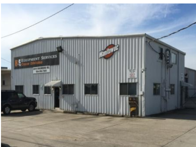
Westbank Warehouse with Yard 2616 ENGINEERS ROAD, BELLE CHASSE
